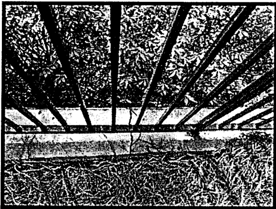
Figure 44 Retaining Wall Crack
